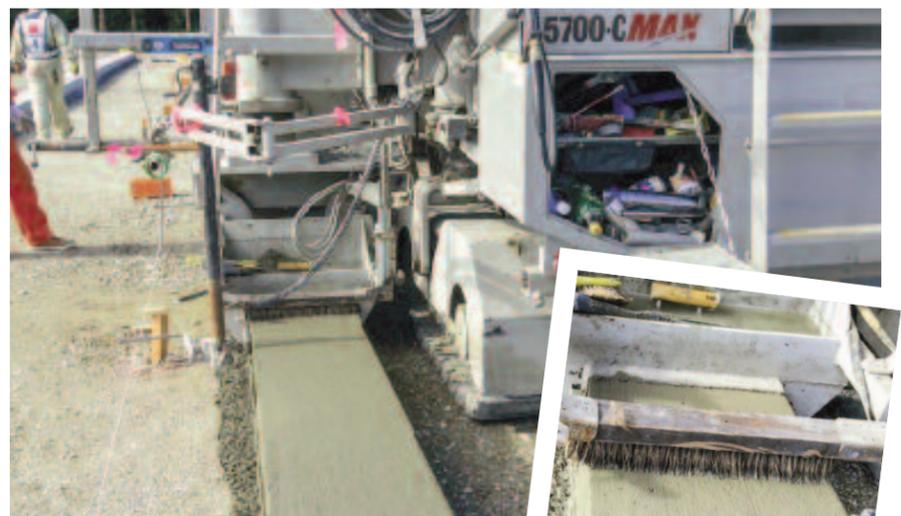
Main: Koyanagawa used their 5700-C-MAX to pour the small profile that the solar panels were then mounted onto.
