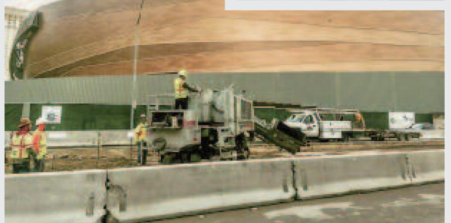
Main: Sahara Concrete's 5700-Super-B rolls onto the jobsite at the new T-Mobile Arena in Las Vegas. Inset: Sahara's crew poured curb in The Park section of the new complex, shown here along the bottom and right side of the photo. (Photo courtesy of Google Images)
