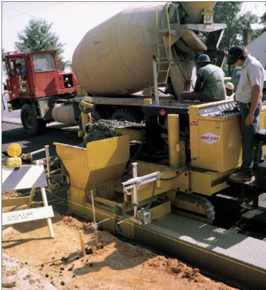
The Curb King 6500, the first slipform paver manufactured by Power Curbers, Inc., was the first machine to pour in the offset position, now an industry standard. The Curb King was the second curb machine that Ken used.
