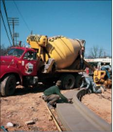
The Power Curber 3000 was the first extruder that Ken used. It poured curb and gutter 33 inches wide (83.8 cm) and had to be lifted by a boom truck on to the tracks that it ran between.
