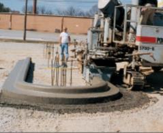
Once the machine is around the curve and comes in contact with the stringline, it is switched from tight radius back to the front-steering sensor. The critical part is when to switch back. If you do it too early it can cause "a dog-leg" in the curb
