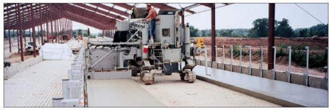
The 8700, in an offset position, rides on the grooved alleys to pour the 7.5-foot-wide beds (2.28 m) for the cows
