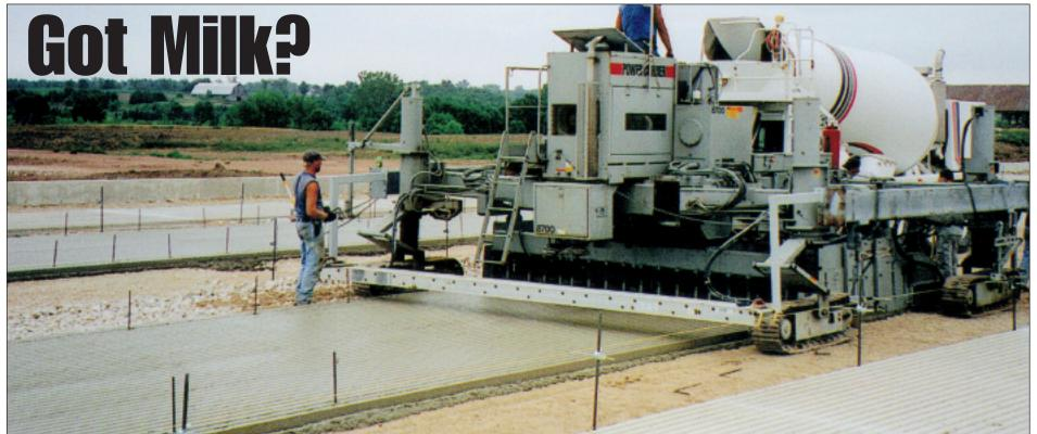
The Power Curber 8700 slipforms grooved alleys that dairy cattle will walk on inside barns in Wisconsin. The grooves help prevent the cows from slipping
