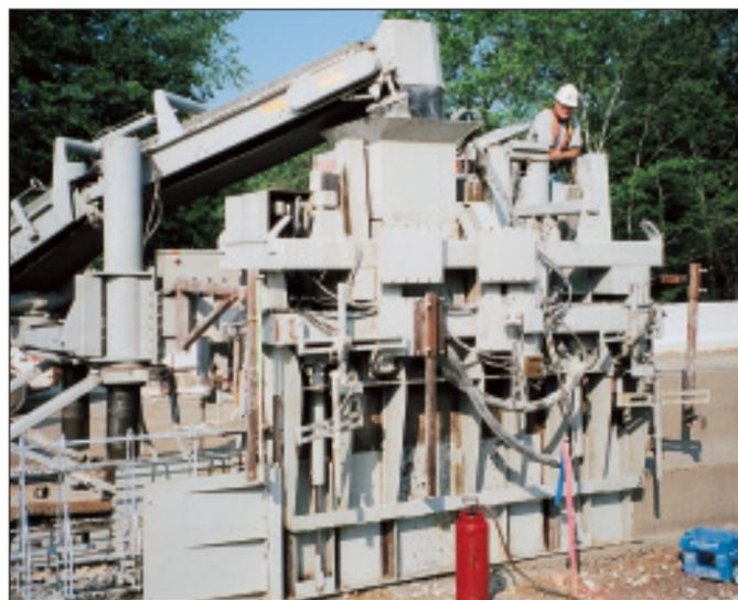
Mold produces barrier that varies in height from 32 to 60 inches (81 to 152 cm)
