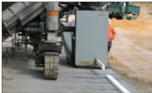
Polystyrene is pushed through the mold to hold the shape of the over-hung lip
