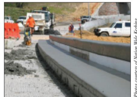
Once the concrete is cured, the polystyrene will be removed, creating the lip for water run-off
