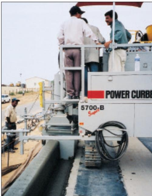
30-inch curb (765 mm) with 10-inch (252 mm) gutter is being poured adjacent to 60 miles (96 kms) of new road in Ranchi
