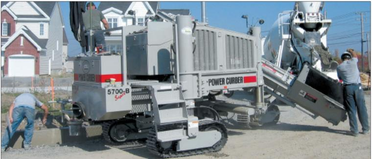
*Ciments Lavallee Ltd. works with 7 slipform machines, including its new SUPER-B, with 80% of the work in curbs and 20% in Jersey barriers*
