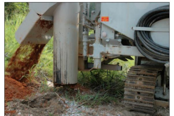
Material in hinged chute is displaced and does not fall back into the pier hole
