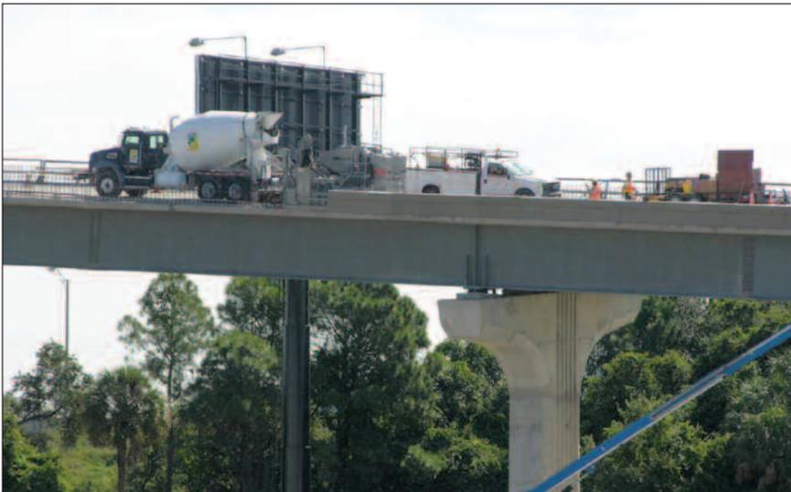
Jeff's Concrete slipforms parapet on ramp leading from Tampa, FL, airport
