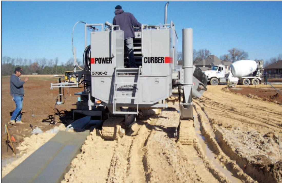
**SUCCESS STORY:** Power Curbers worked with Custom Curb & Edging, widening the tracks on the front and left crawlers to 16 inches (40.6cm) to keep the machine from bogging down in soft soil and delaying production
