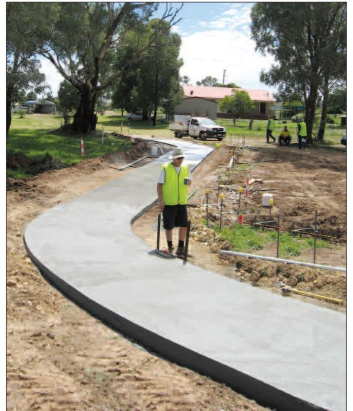
Malvick Constructions of Bathurst, New South Wales, Australia, poured this 6.5-foot foot path (2 m) in Orange, Australia, located in central New South Wales, with the Power Curber 5700-C.
