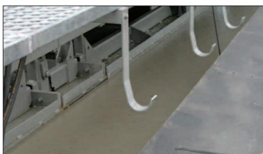
High-quality concrete product directly behind machine, requiring very little finishing with belt finisher or burlap drag
