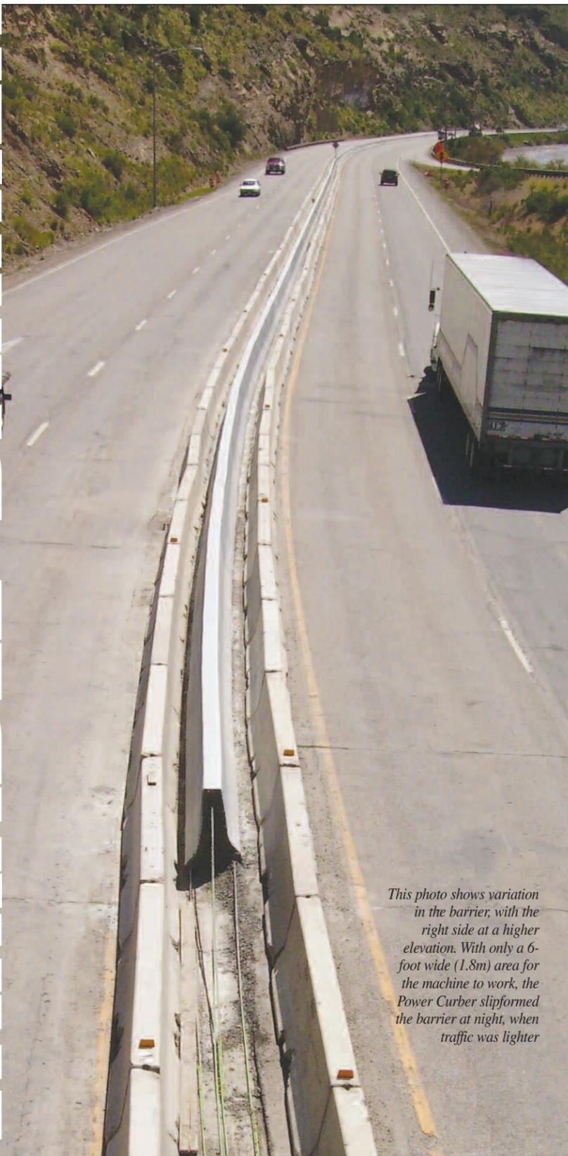
*This photo shows variation in the barrier, with the right side at a higher elevation. With only a 6-foot wide (1.8m) area for the machine to work, the Power Curber slipformed the barrier at night, when traffic was lighter*
