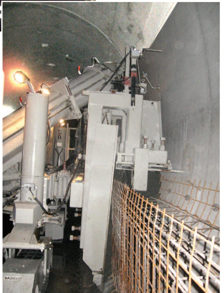
The custom built mold has to adjust to the varying tunnel diameter and accommodate the steel reinforcement.
