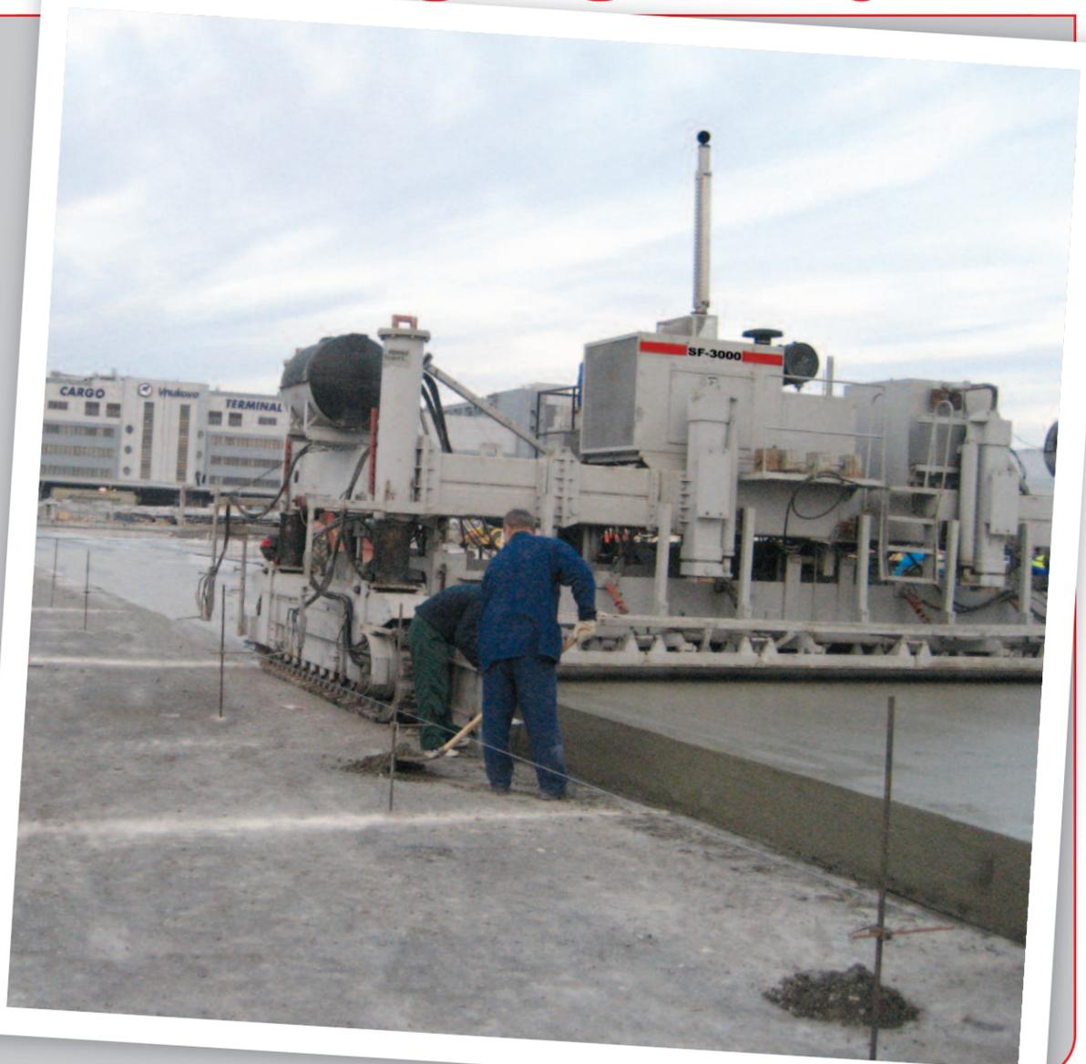
*Power Pavers SF-3000 paving 16" (40cm) thick slab at Moscow airport.*
