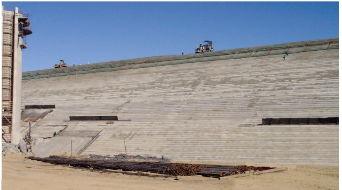
The Power Curber poured 103 passes across the face of the 165 ft. (50m) tall dam.
