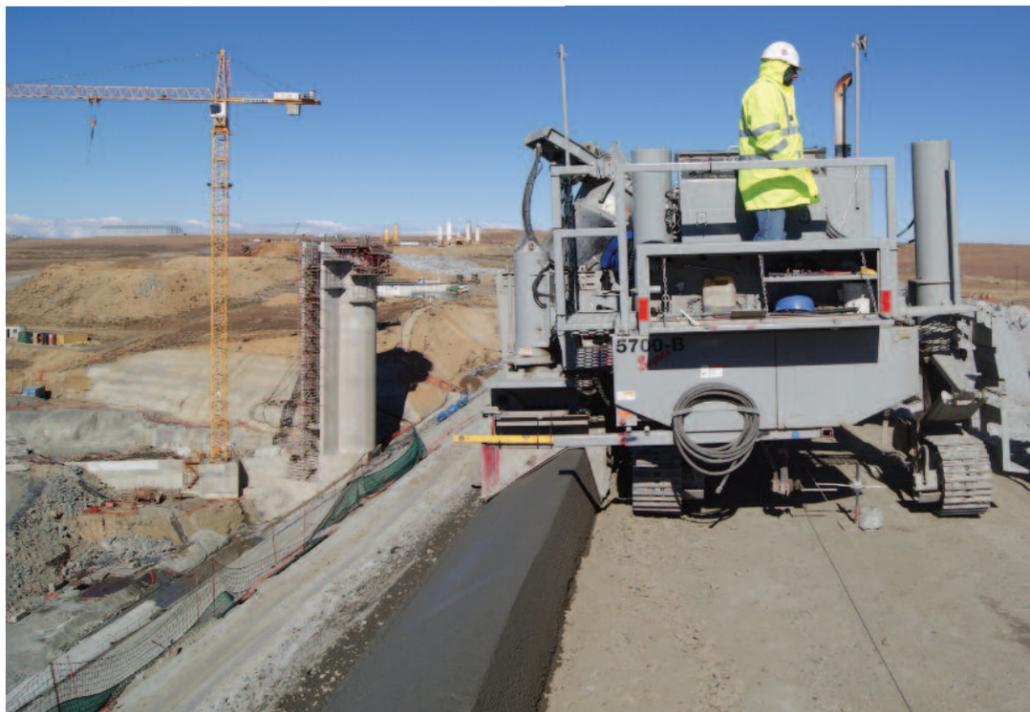
For each layer, the trapezoidal curb is poured first. Then, rock backfill is placed and compacted behind the curb.
