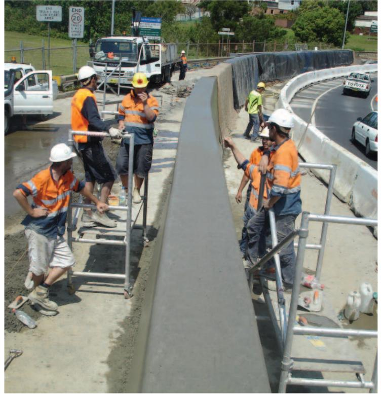
Due to the height of the wall, the finishing crew required scaffolding for their work.
