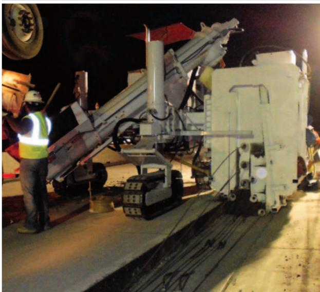
Rebar is fed into the wall through ports at the front of the mold.
