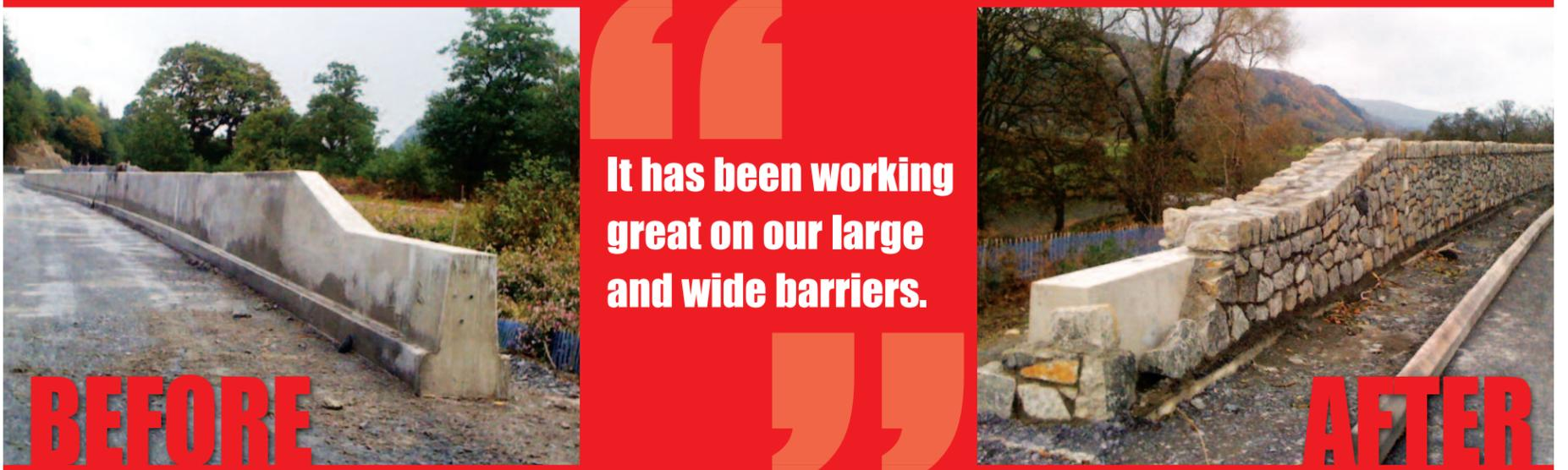
Before and after photos of slip-formed barrier with natural stone facing.
