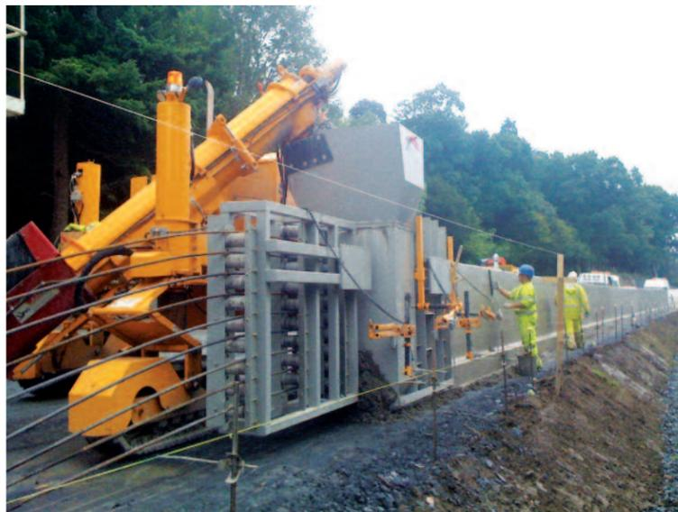
5700-C-Max with barrier mold and rebar feeder pouring in the UK.
