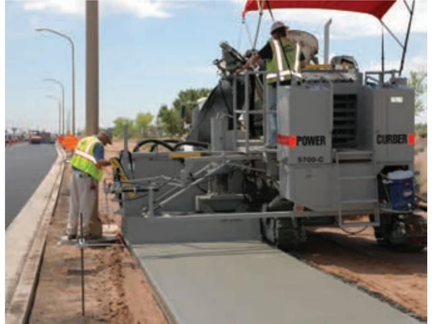
Wayne Irby from Power Curbers’ product support team offers guidance and know-how to Albuquerque Asphalt’s machine operator as the 5700-C pours a clean, smooth 6’ sidewalk.
