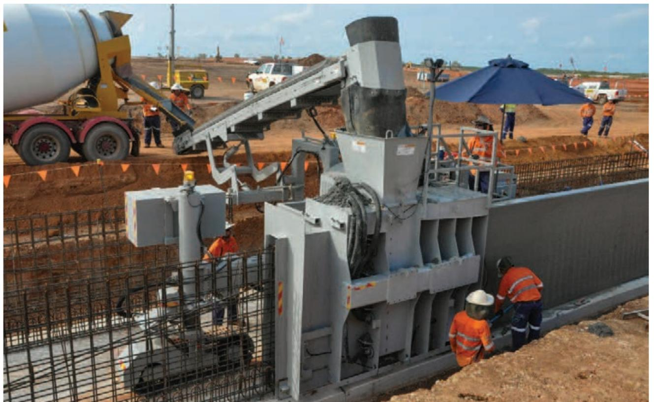
The 5700-C-MAX was heavy enough to wield enormous custom molds for smooth pours, but was also compact enough to fit inside the canal to pour the side walls.
