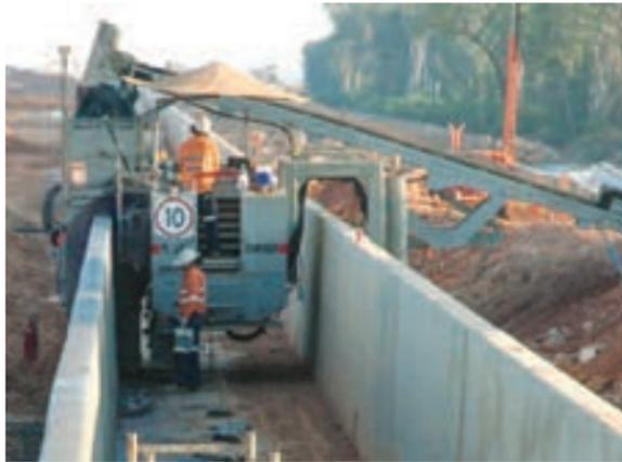
**W**hen Australian firm Baldwin Civil NT was approached about constructing a regulating reservoir as part of the new Inpex natural gas project in the Northern Territory, they didn't even know if it was possible to slipform a 2.1 m (6 ft 10 in) high wall.
