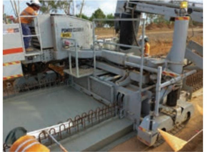
Top Left: Brothers John and David Baldwin met the challenge of the massive walls required for the canal with their custom-engineered Power Curber 5700-C-MAX machines.
