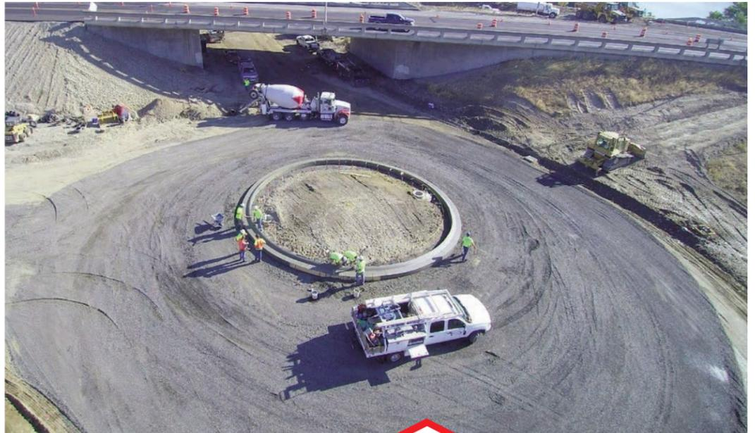
*Knox Concrete was able to minimize manual finish work on the roundabouts due to the flexibility of their 5700-B*
