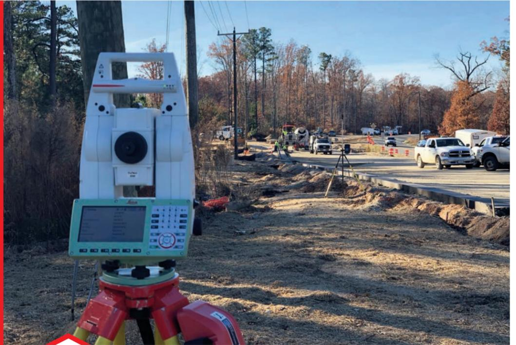
*Using a Leica system allows the Power Curber to stay accurate even when working around tall trees*
