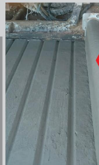
*JKL Construction using their Power Paver SF-2700 to slipform a grooved cattle barn floor*
