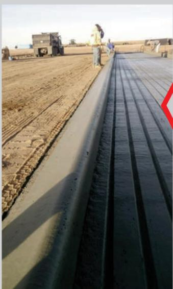
*This slipform design produced by the Power Paver paving kit will help contain the cattle waste and facilitate easy flushing and cleaning due to the longitudinal grooves*
