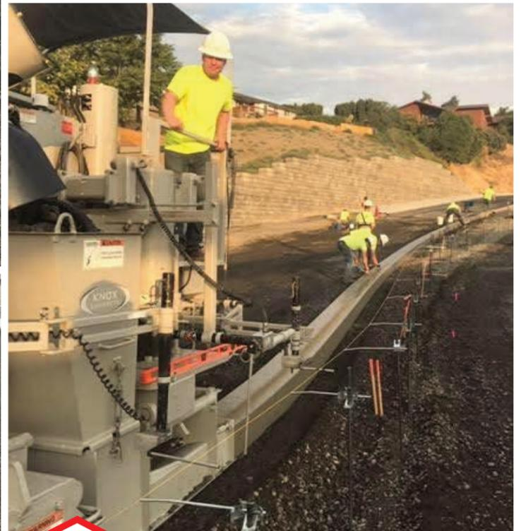
*Knox Concrete slipforming roll curb on a ramp with their 5700-B*
