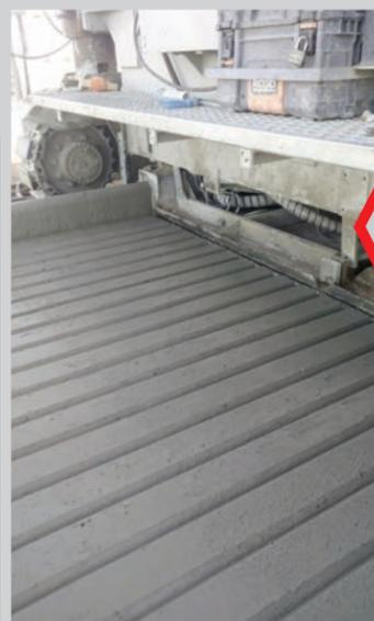
*The paving kit on the Power Paver SF-2700 is able to include the floor and integrated curbs on both sides all in one pass, saving time and money*
