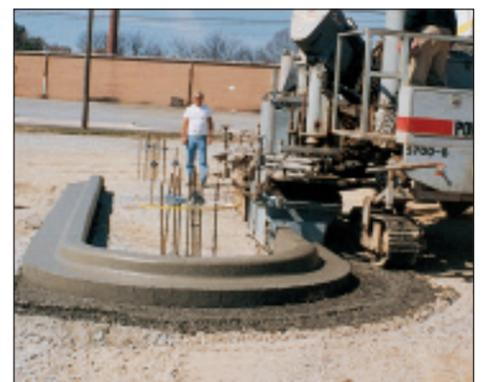
Once the machine is around the curve and comes in contact with the stringline, it is switched from tight radius back to the front-steering sensor. The critical part is when to switch back. If you do it too early it can cause "a dog-leg" in the curb
