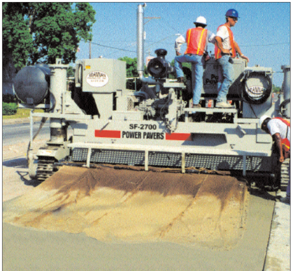
The 2700 paves up to 27 feet wide (7.32 m), and with extensions, up to 32 feet wide (9.75 m)
