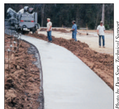
Here's another sidewalk application. This 5-foot (1.52m) walk was poured by McManus Construction in Lake Charles, LA.
