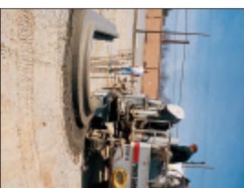
Most contractors consider tight radius the most difficult part of curb-and gutter work. But once you've mastered it, you'll save a lot of labor. There will be just a few feet of handwork to do on the straight ways.
