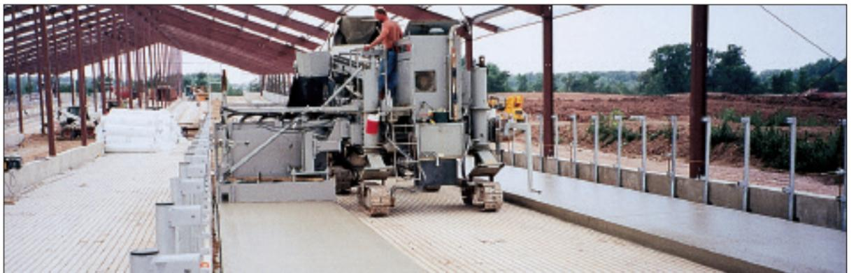
The 8700, in an offset position, rides on the grooved alleys to pour the 7.5-foot-wide beds (2.28 m) for the cows
