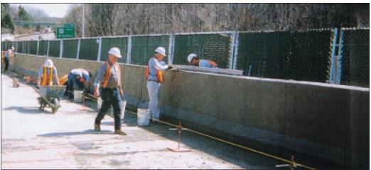
Dirigo added 4 inches to the bottom of the mold to adjust for the grade difference
