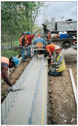
The 5700-B (with seat added by NESC) slipforms footer for MSE wall as part of same project
