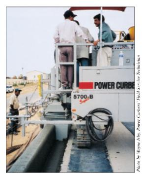
30-inch curb (765 mm) with 10-inch (252 mm) gutter is being poured adjacent to 60 miles (96 kms) of new road in Ranchi
