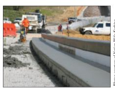
Once the concrete is cured, the polystyrene will be removed, creating the lip for water run-off
