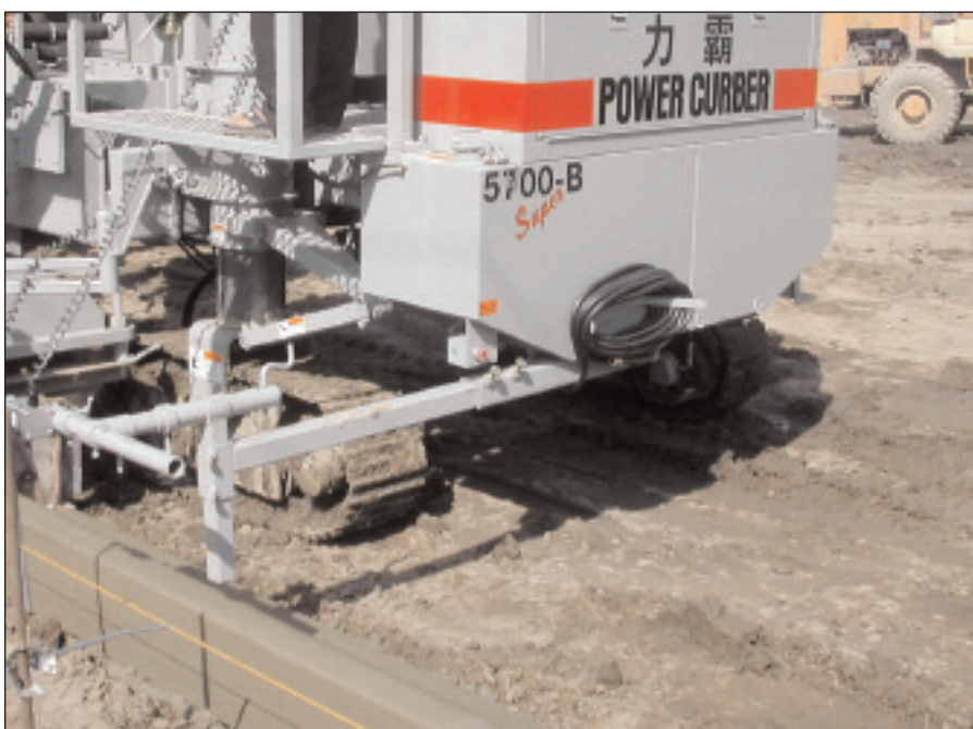
Curb and gutter being slipformed as part of Zhangjinkou Highway Project
