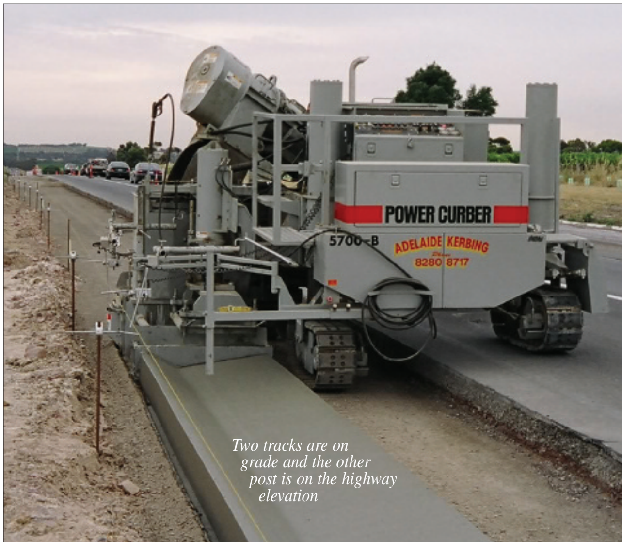
The machine is positioned on edge of existing pavement, in preparation for bringing the right rear post off the pavement and down a ramp that the crew constructed, while continuously pouring
