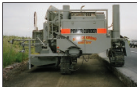
The machine is positioned on edge of existing pavement, in preparation for bringing the right rear post off the pavement and down a ramp that the crew constructed, while continuously pouring
