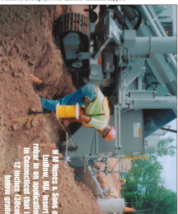
H M Nunes & Sons of Ludlow, MA, inserts rebar in an application in Connecticut that is 12 inches (30cm) below grade.
