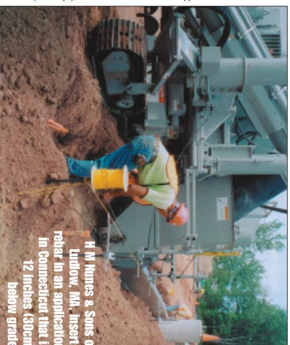
H M Nunes & Sons of Ludlow, MA, inserts rebar in an application in Connecticut that is 12 inches (30cm) below grade.
