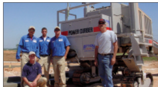
Action Concrete's curb crew with Phil Myers, right, Power Curbers' service manager in Georgia, Alabama and east Tennessee. Crew members are, left to right, Louis Fernandez, Brian McConnell and Adam Ellis. Michael Smith, supervisor of the curb crews, is kneeling
