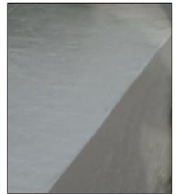
*Exact match-up between side forms and paving pan result in a product with a crisp, sharp edge*
