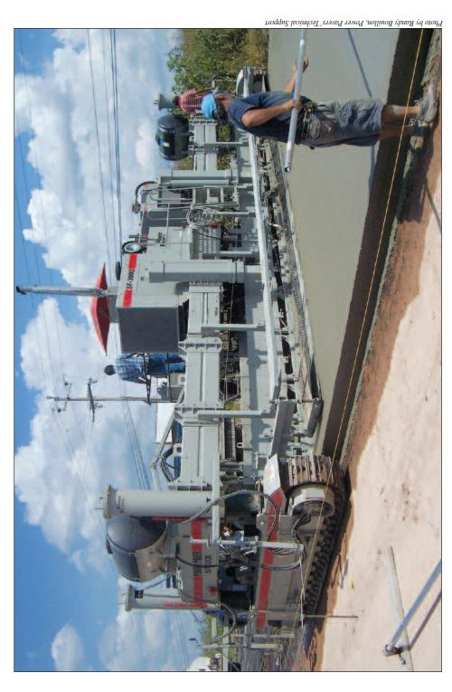
A concrete highway built outside the city of Zapotlanejo, Guadalaform machine, and a TC-2700 by Power Pavers, that was used to cure jara, Mexico, involved an SF-3000 by Power Pavers, a two-track slipthe concrete and add texture for rideability. The road is 34 feet wide
