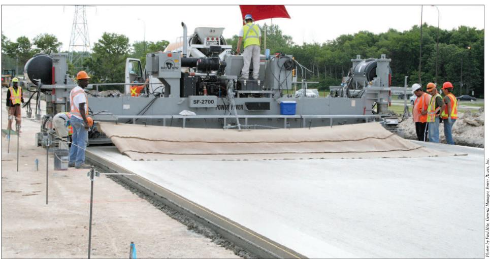
The SF-2700 paves 27 feet (8.3 meters) wide on Bishop Gerandin Boulevard in Winnipeg, Manitoba. The project, on a street with a traffic volume of up to 80,000 cars per day, requires 5 different paving widths
