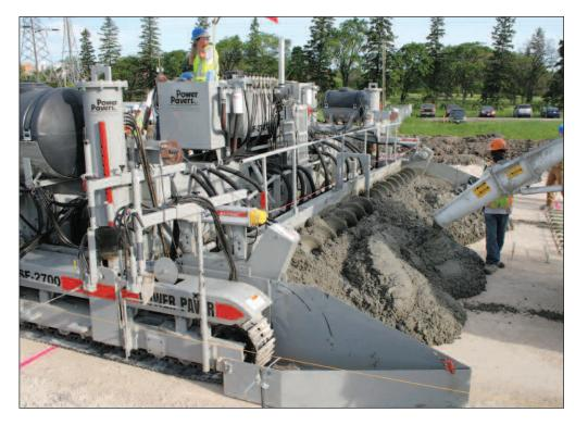
of concrete and was slipformed in 7 hours. "We averaged 78 cubic meters (839 cu ft) an hour," John says.
