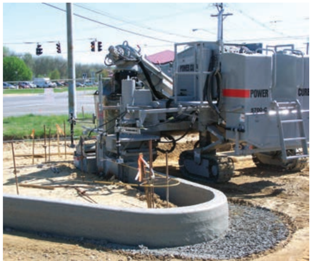
Tight radii are all in a day's work with Curbs Etc's 5700-C.
