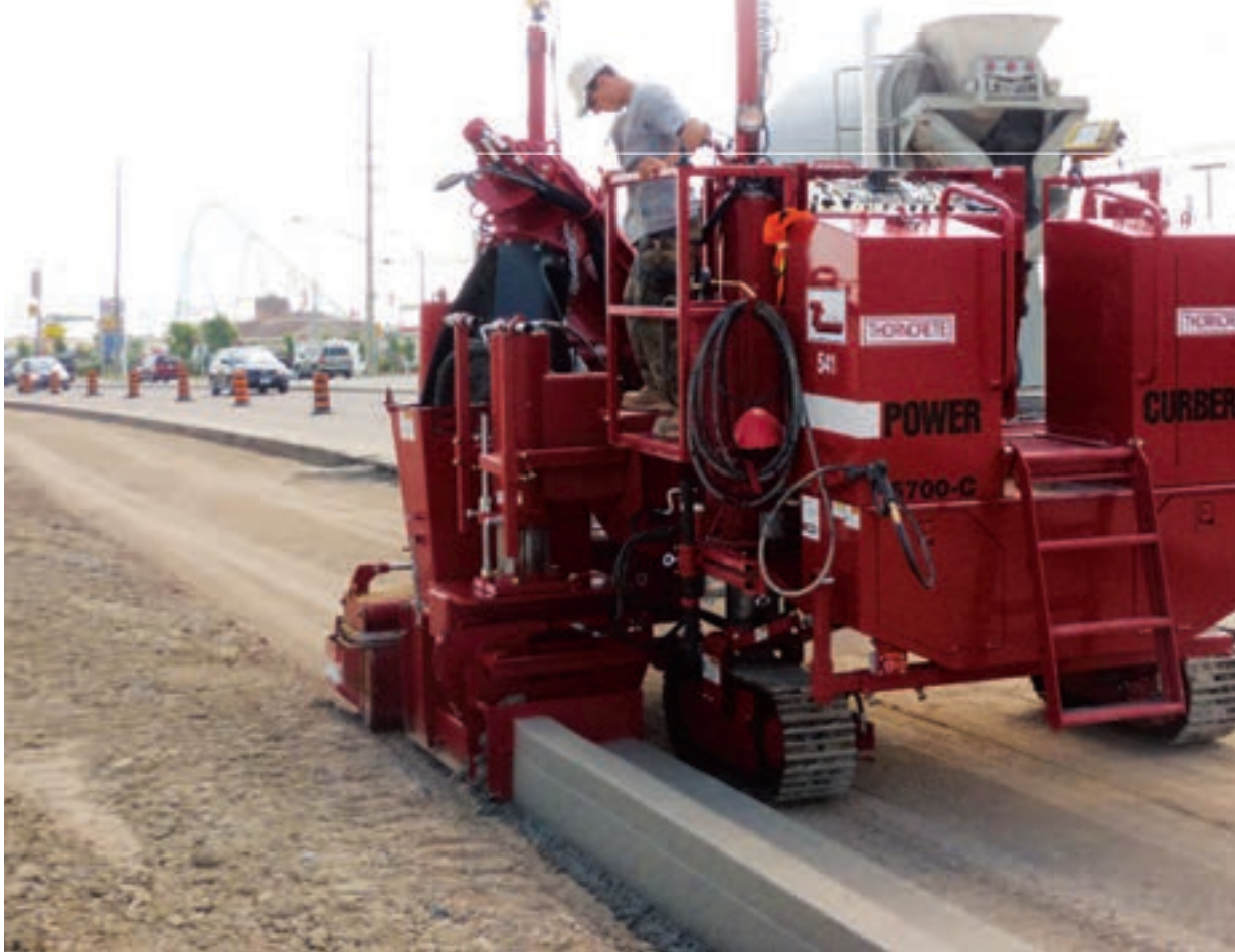
Above: 5700-C, with Topcon Millimeter GPS controls, pouring without stringline in Toronto. Inset: Smooth and straight, and no stringline to set and take down.
