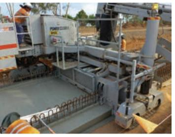
Top Left: Brothers John and David Baldwin met the challenge of the massive walls required for the canal with their custom-engineered Power Curber 5700-C-MAX machines.
