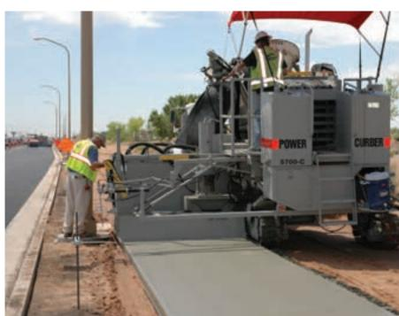
Wayne Irby from Power Curbers' product support team offers guidance and know-how to Albuquerque Asphalt's machine operator as the 5700-C pours a clean, smooth 6' sidewalk.
