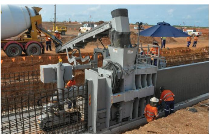
The 5700-C-MAX was heavy enough to wield enormous custom molds for smooth pours, but was also compact enough to fit inside the canal to pour the side walls.
