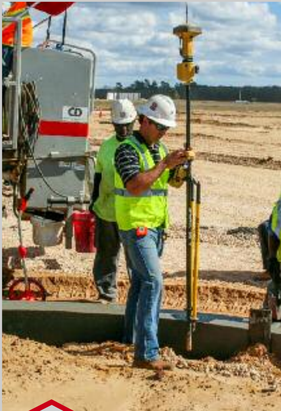
Owner Jacob Cunningham checks the accuracy of the curb placement with the Topcon rover. Photo by Larry Trojak, Trojak Communications
