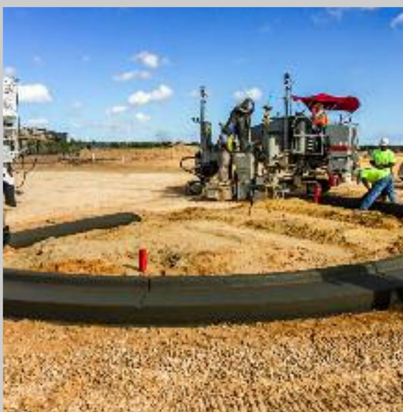
Owner Jacob Cunningham checks the accuracy of the curb placement with the Topcon rover. Photo by Larry Trojak, Trojak Communications
