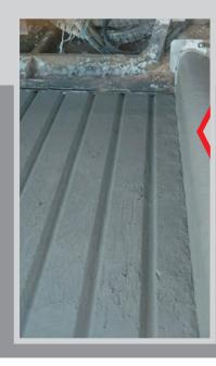
JKL Construction using their Power Paver SF-2700 to slipform a grooved cattle barn floor
