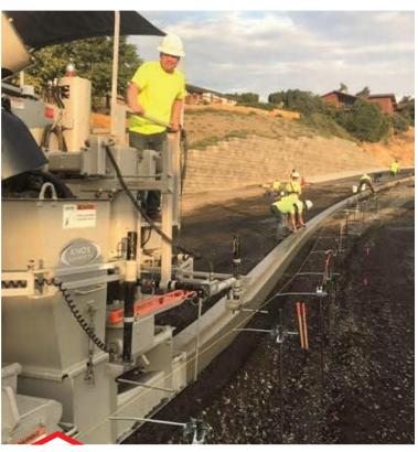
Knox Concrete slipforming roll curb on a ramp with their 5700-B
