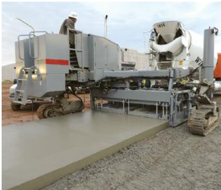
Center pour paving 10' (3m) wide. Concrete is dumped directly into a hopper at the front of the paving mold.
