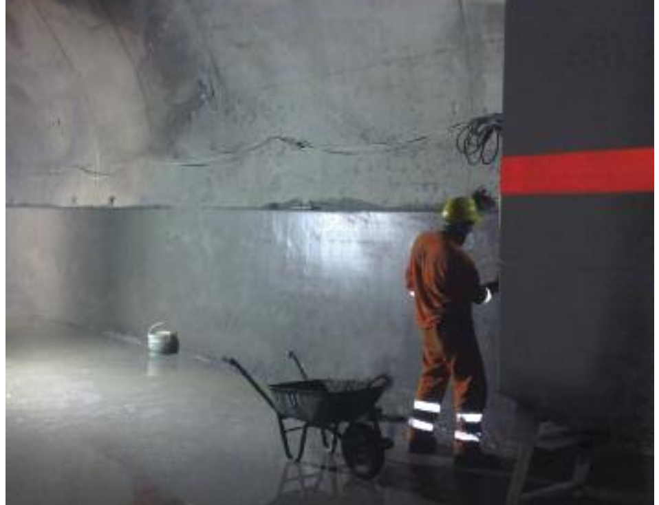
Platform & wall structure poured along a tunnel wall – mold is adjustable in height and width to accommodate varying tunnel diameter.
