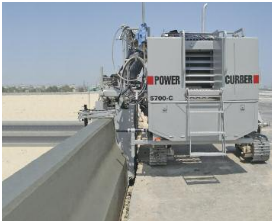
Barrier poured below grade, 49" (1.25m) tall.
