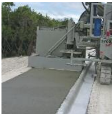
Sidewalk adjacent to back-of-curb. Sensing off-curb.
