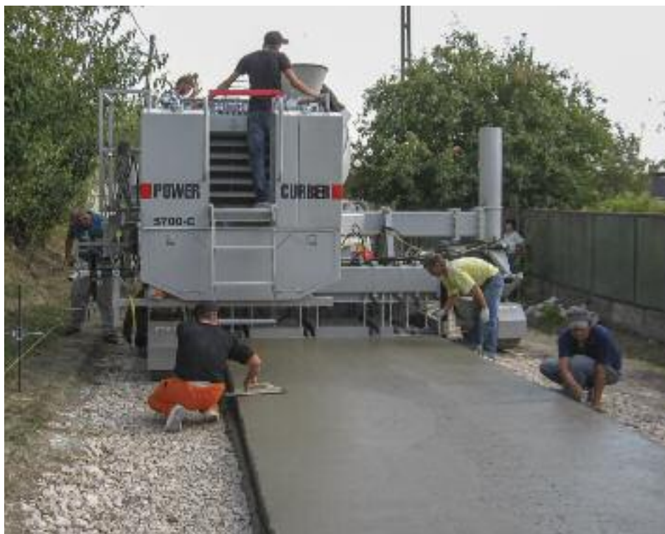
Paving 10' (3m) wide in Romania. Center pour paver is sectional for varying paving widths.
