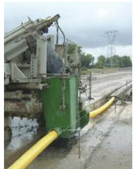
Slotted drain showing inflated tube.
