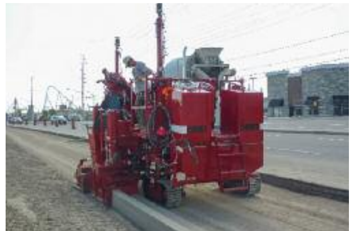
Pouring curb & gutter with 3-D (stringless) control.
