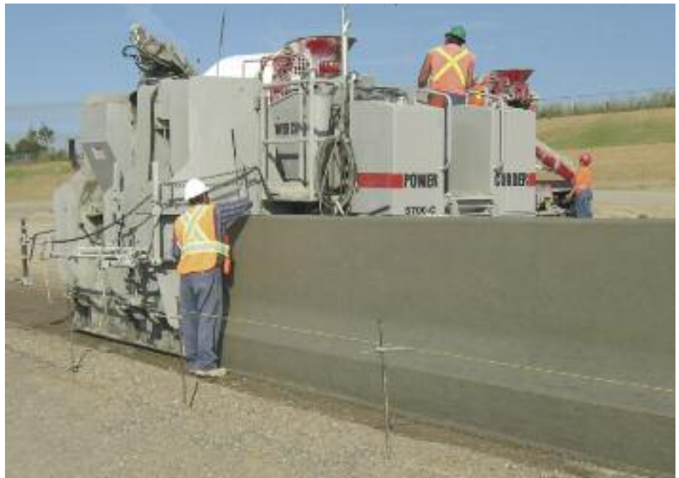
Variable barrier, up to 68" (1.72m) tall in Ontario.
