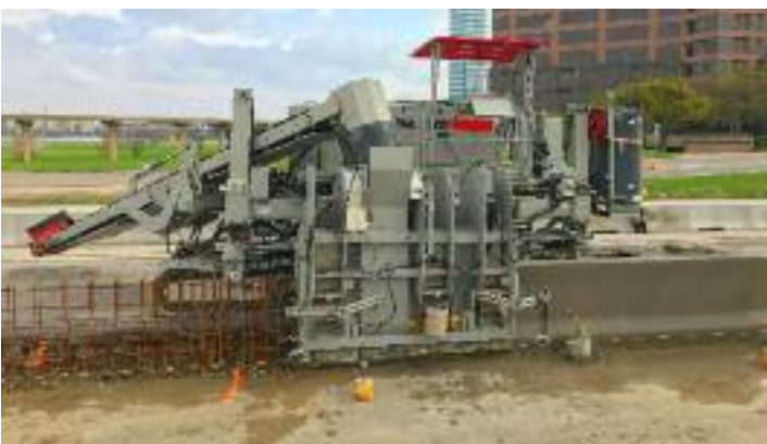
▲ Power Curbers 7700 Multipurpose Slipform Machine Pouring Barrier
