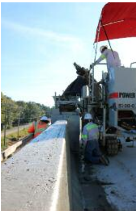
5700-C pouring bridge parapet in North Carolina.
