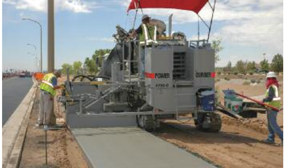
Pouring a 6' sidewalk with minimal side clearance.
