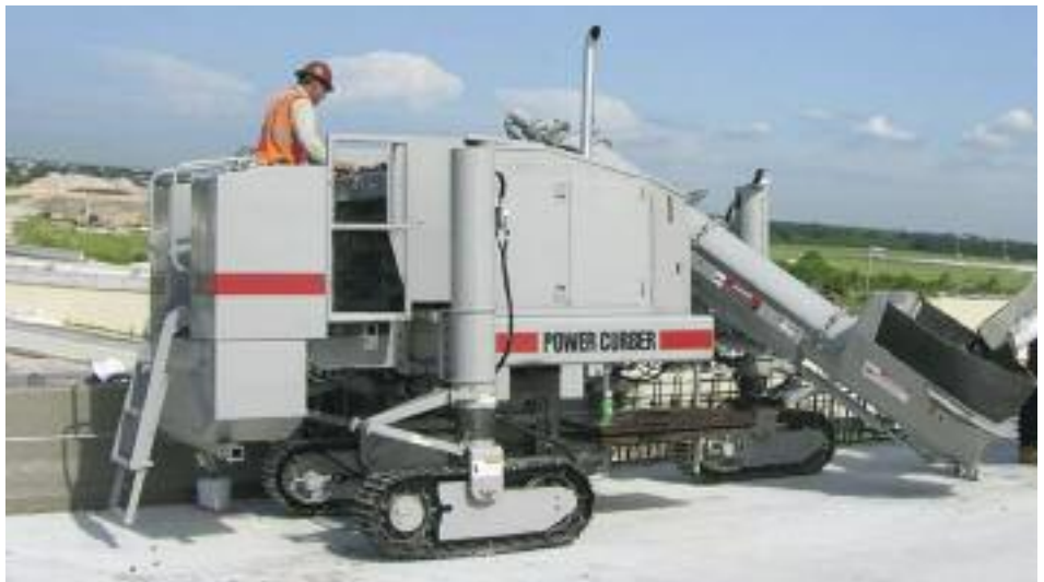
5700-C pouring bridge parapet in Florida.
