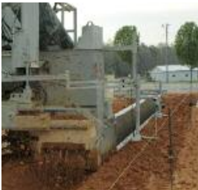
Custom trencher trimmer and poultry house foundation.
