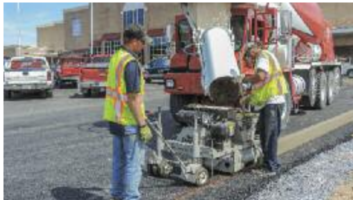
▲ Power Curbers 150 Extruded Curb Machine
