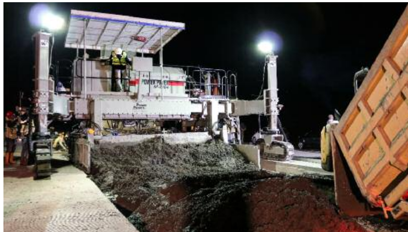
An SF-2404 paving a highway
