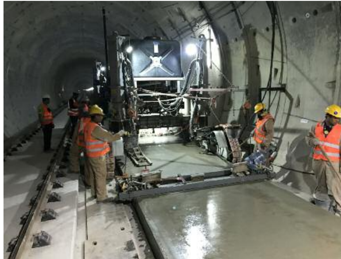
An SF-2404 slipforming railway
