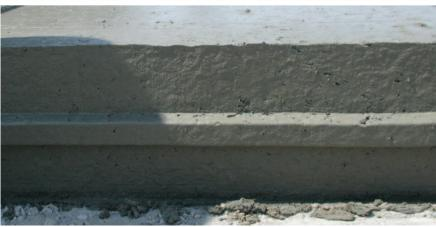
Edge of pavement with optional key-way inserter (top), and optional male key-way block-out (bottom).
