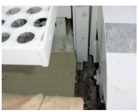
The side-forms are connected to the tracks.
