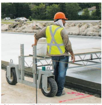
Optional non-powered WB-2700 Work Bridge gives the crew access to the slab.
