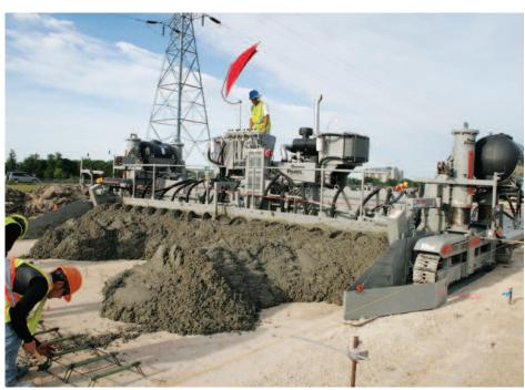
Front view of the SF-2700 paving over dowel baskets in Saskatchewan.
