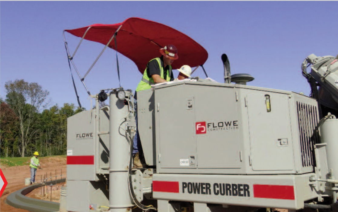
M.O. Flowe pouring 48” curb & gutter with a Power Curber 5700-C.
