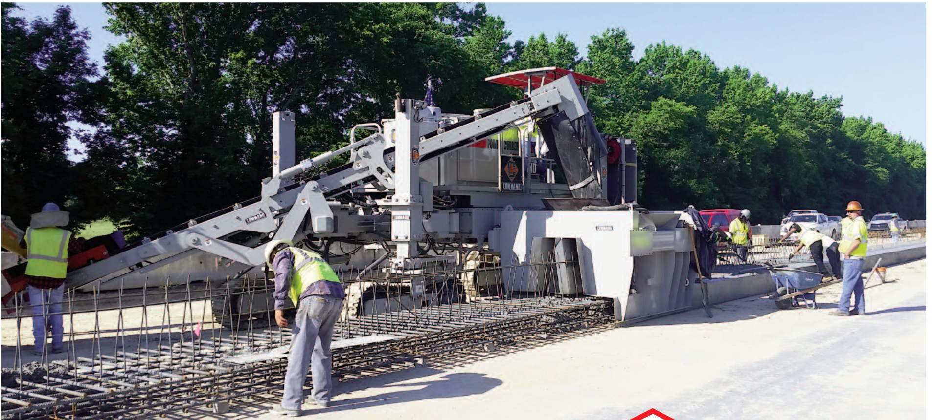
Command's 7700 using a custom mold to pour barrier foundation
