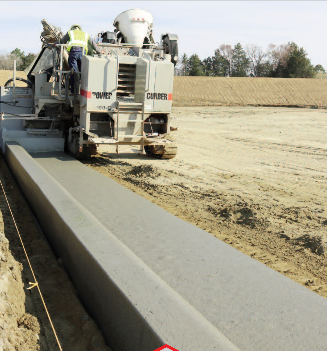
M.O. Flowe pouring 48” curb & gutter with a Power Curber 5700-C.
