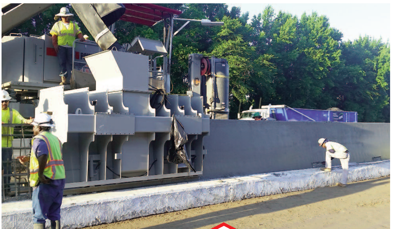
54” barrier slipformed on top of the foundation
