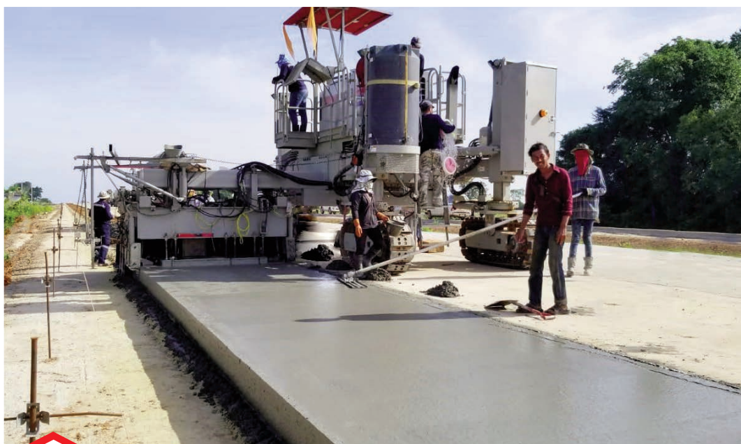
A 7700 paving a 2.5 meter (eight-foot) wide shoulder in the offset position.
