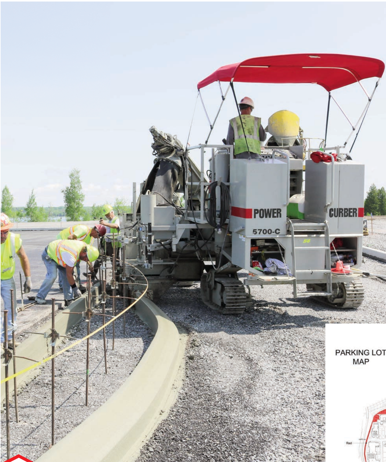
JJP Slipforming a unique semicircle-shaped island
