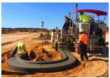
Pouring curb & gutter with 3-D (stringless) control.
