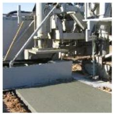
Sidewalk adjacent to back-of-curb. Sensing off-curb.
