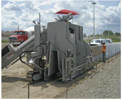
MAX package pouring large variable barrier wall.
