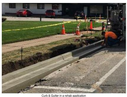
Tapered curb & gutter, poured over dowels adjacent to the pavement.
