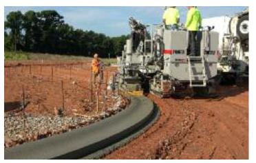
The rear post on the 5700-D-MAX can be returned to its standard position for pouring curb and gutter.
