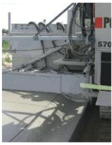
Monolithic curb, gutter, and sidewalk.
