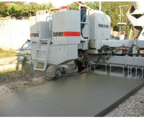
Paving 10' (3m) wide. Center pour paver is sectional for varying paving widths.
