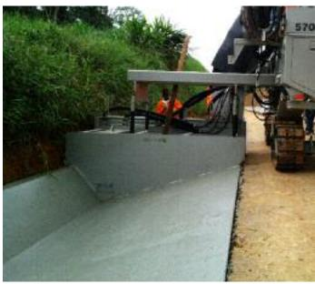
V-Ditch in Equatorial Guinea, 7' (2.2m) wide and 18" (.45m) deep, poured adjacent to pavement.
