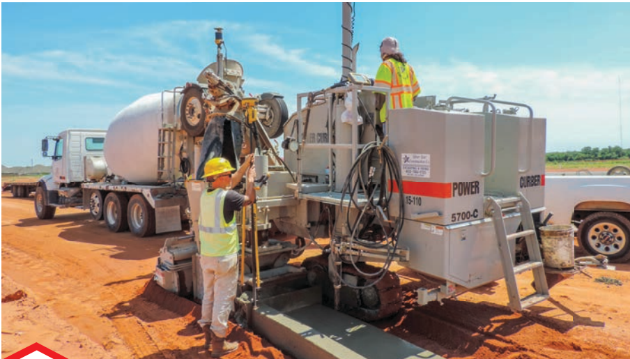
A member of Silver Star's crew uses the Topcon rover to check the accuracy of the curb.
