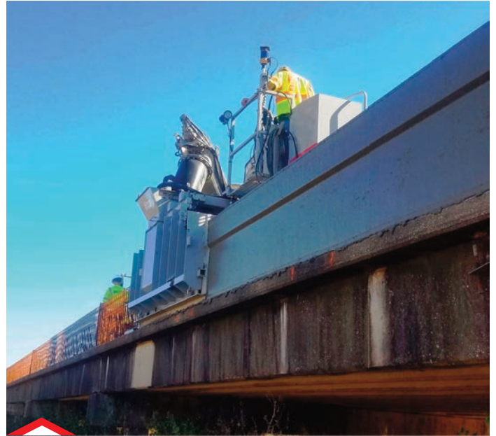
Texas bridge parapet installed with a Power Curber 5700-C using Topcon controls.
