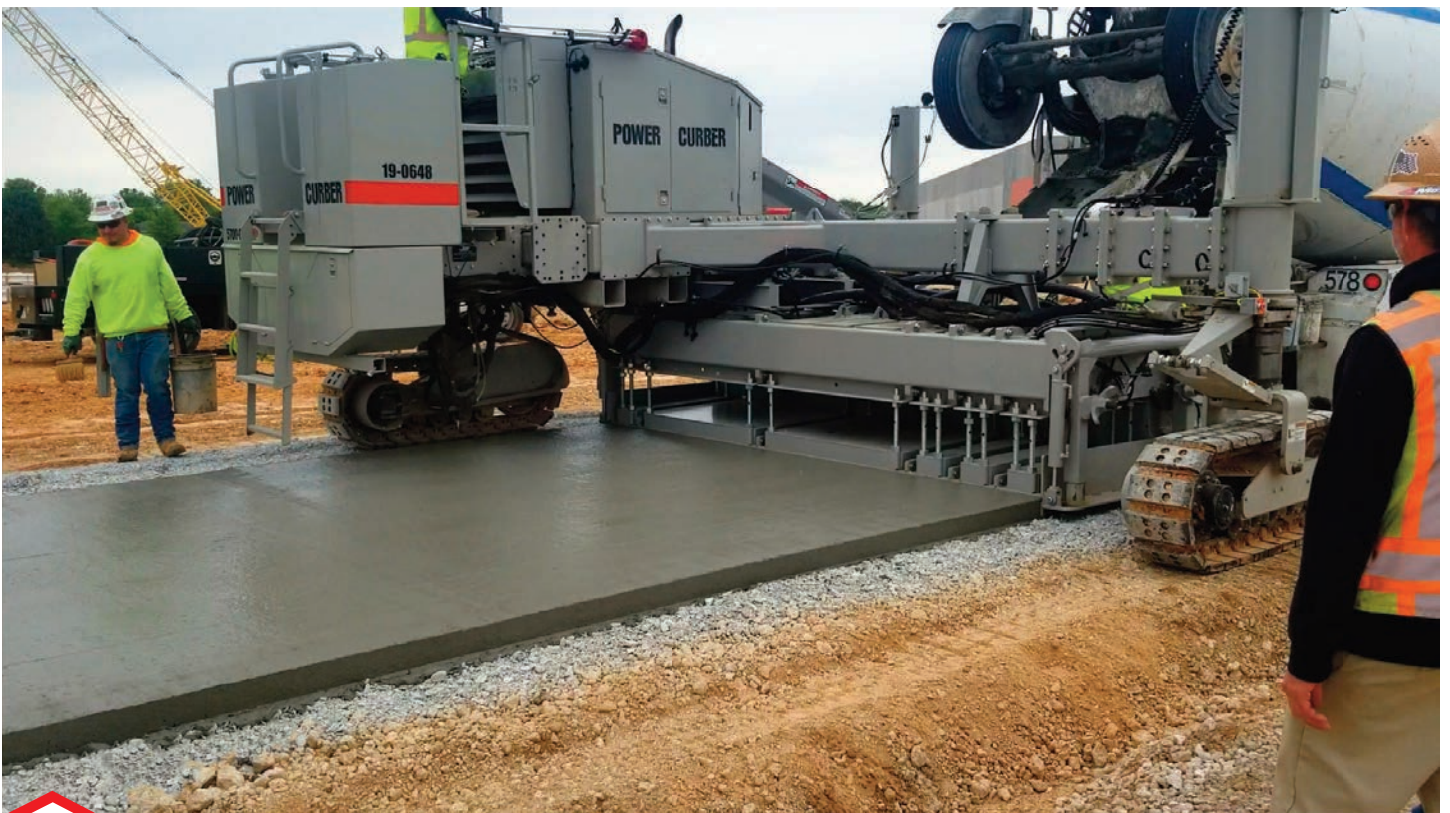
This 5700-C-MAX is set up in a centerpour configuration and pouring dolly pads with a Topcon mmGPS system in Kansas.
