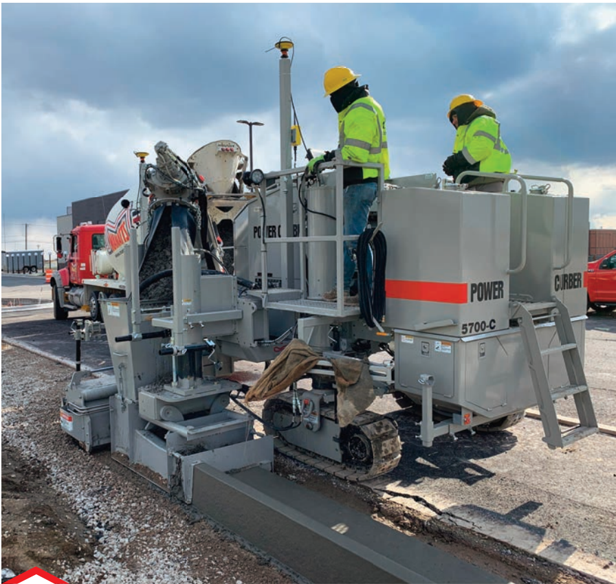
This 5700-C equipped with Leica controls is slipping below grade in Illinois.
