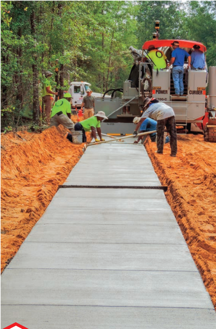
3D system used in Alabama around dense tree cover.
