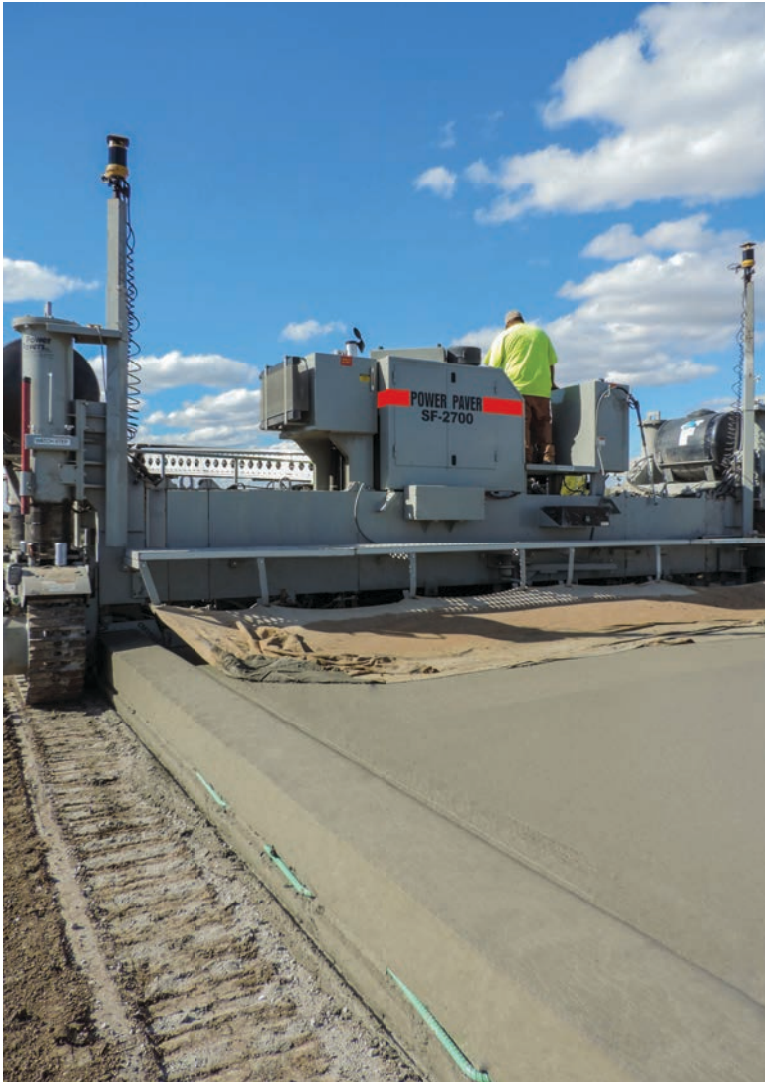
Highway paving with a Power Paver SF-2700 and Trimble control system in Florida
