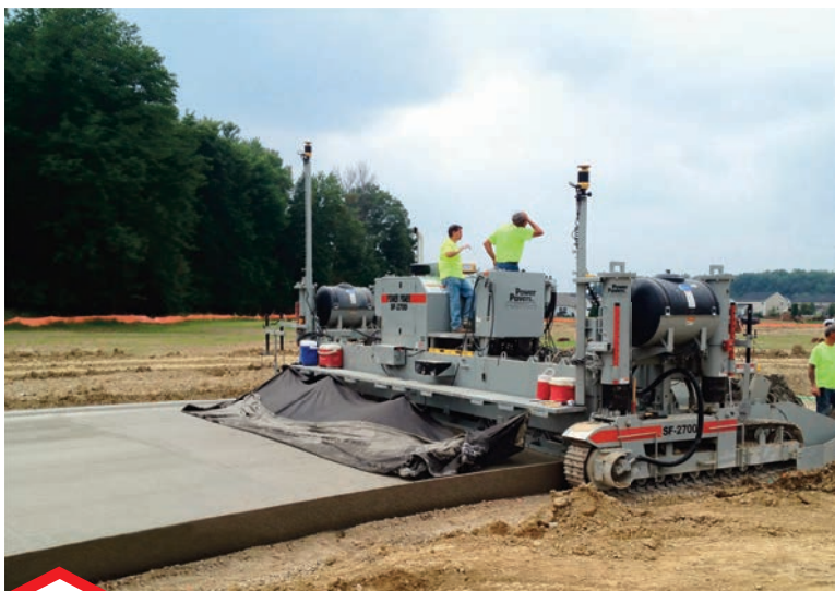
This SF-2700 using a Topcon system is pouring the pavement and integral curb for both sides of an Ohio housing development street in one pass.
