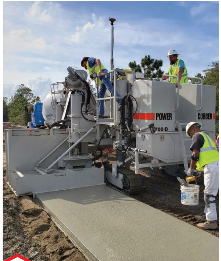
The 5700-D pouring sidewalk with a Leica system in Florida. The latest model is more responsive than ever and the 3D providers love how well it works with their systems.
