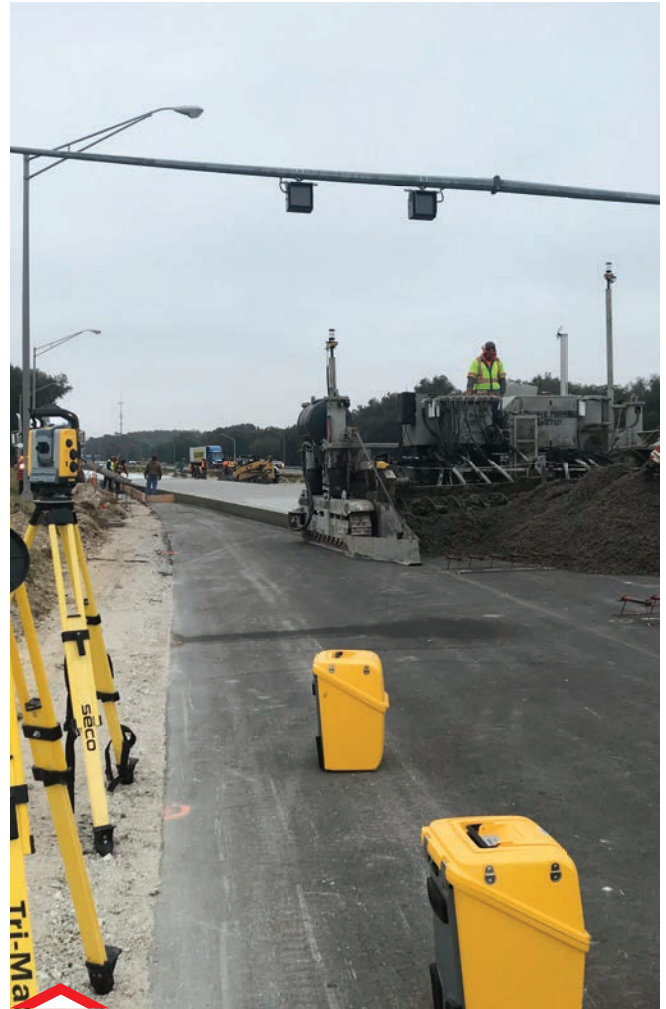
Highway paving with a Power Paver SF-2700 and Trimble control system in Florida
