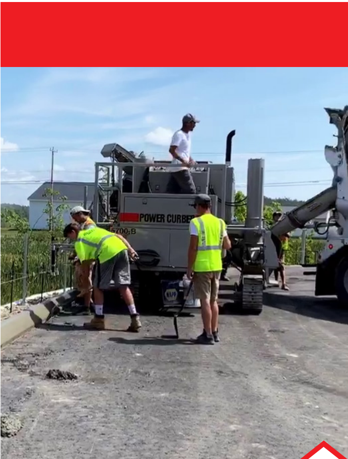
Associates of Williams Brothers Construction, Inc. install curb
