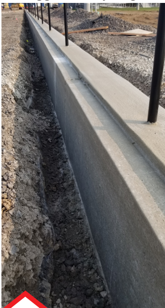
Slipforming this job saved Millennium Construction about a month vs hand forming
