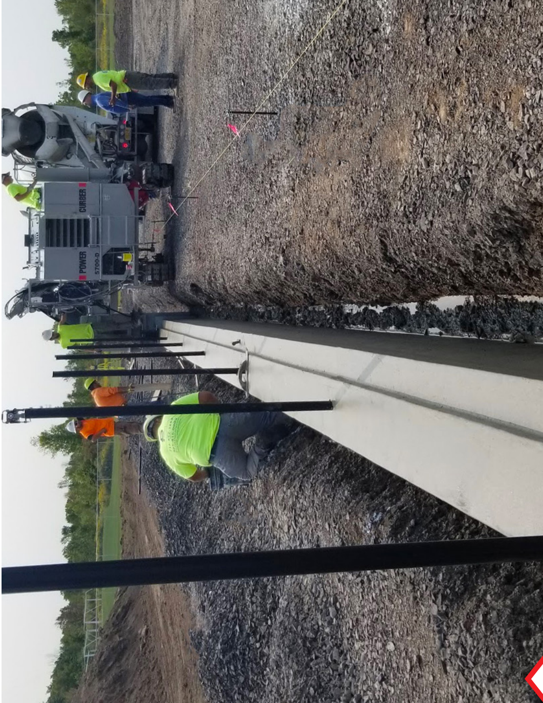
Dual-purpose fence foundation/turf anchor slipformed below grade
