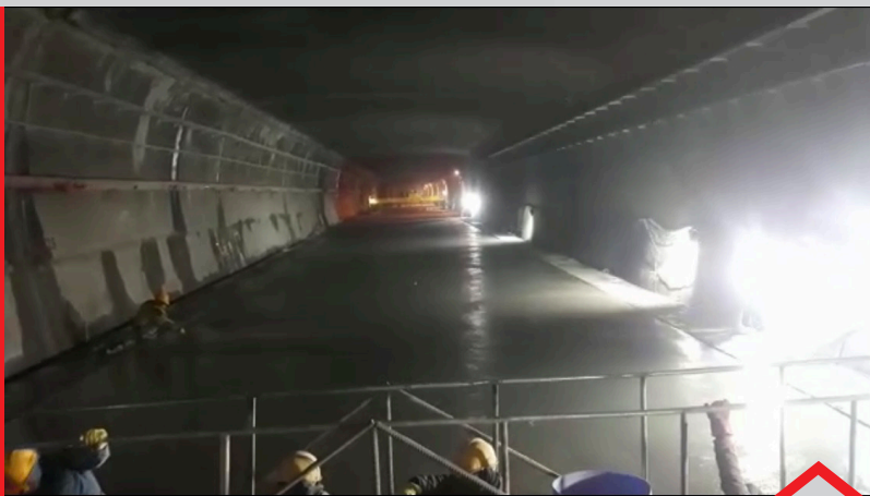
The Power Paver SF-2700 was perfect for paving the Atal Tunnel due to minimal side clearance requirements
