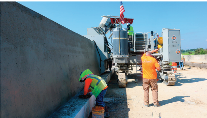
▲ Power Curbers 7700 Multipurpose Slipform Machine Pouring Variable Barrier
