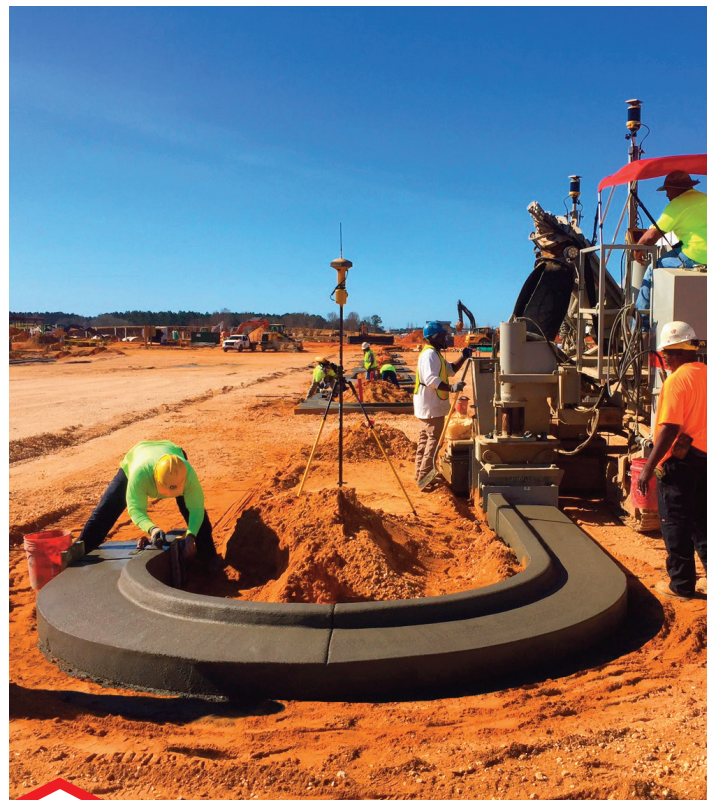
In this Alabama parking lot with many tight-radius islands, avoiding tricky string-line setup saved many hours.
