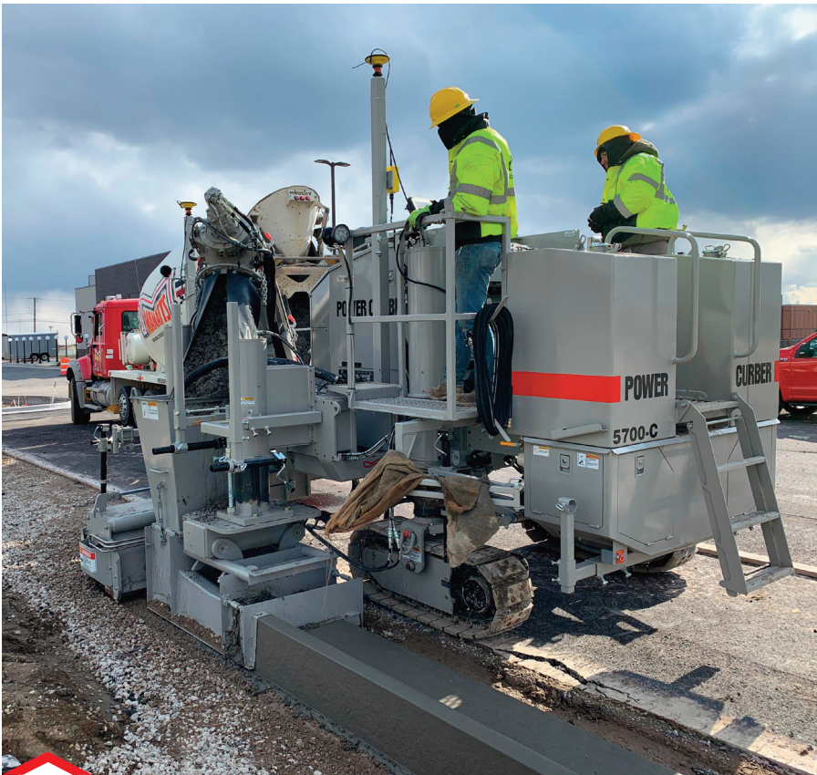
This 5700-C equipped with Leica Geosystems controls is slipping below grade in Illinois.
