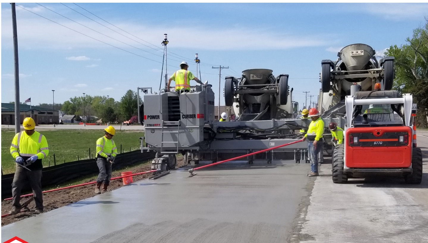
This 5700-D-MAX in centerpour configuration is pouring a highway lane addition with Trimble guidance in South Dakota.
