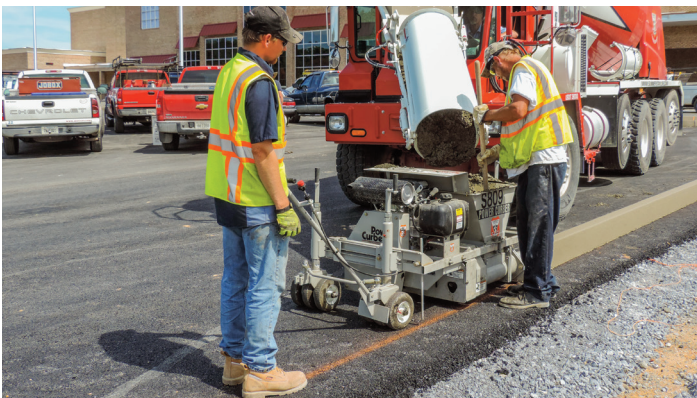
▲ Power Curbers 150 Extruded Curb Machine
