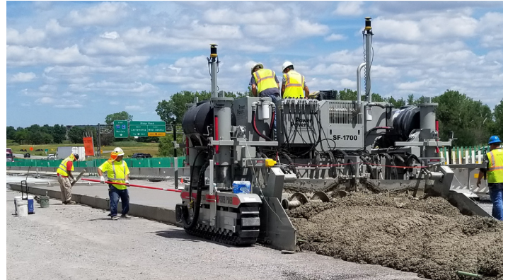
▲ Power Pavers SF-1700 and SF-2700 Slipform Pavers (Optional Topcon)
