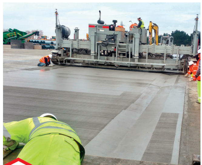
This SF-3000 is using a Trimble system to pave a port storage pad with a shallow ditch in the United Kingdom.
