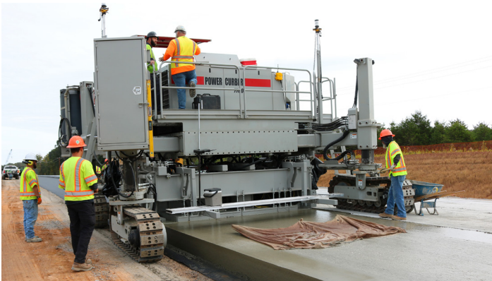
▲ Power Curbers 7700 Multipurpose Slipform Machine Paving (Optional Trimble)
