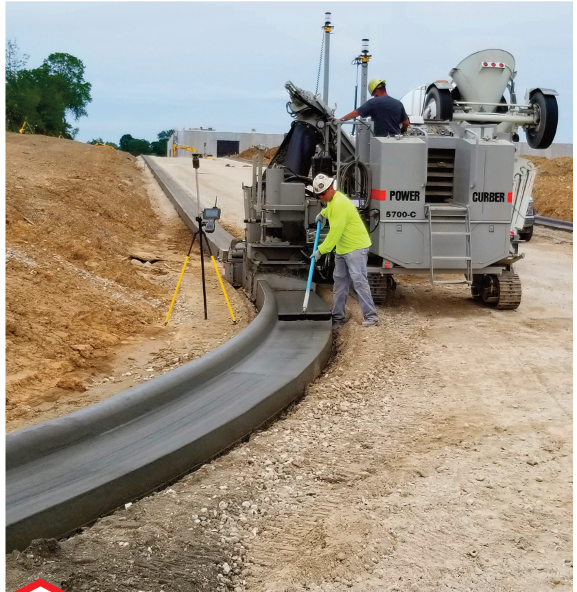
An Ohio crew using a 5700-C outfitted with Trimble controls wrapping up their very first pour with a 3D system.
