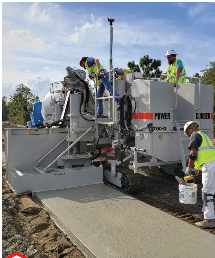
The 5700-D pouring sidewalk with a Leica Geosystems system in Florida. The latest model is more responsive than ever and the 3D providers love how well it works with their systems.
