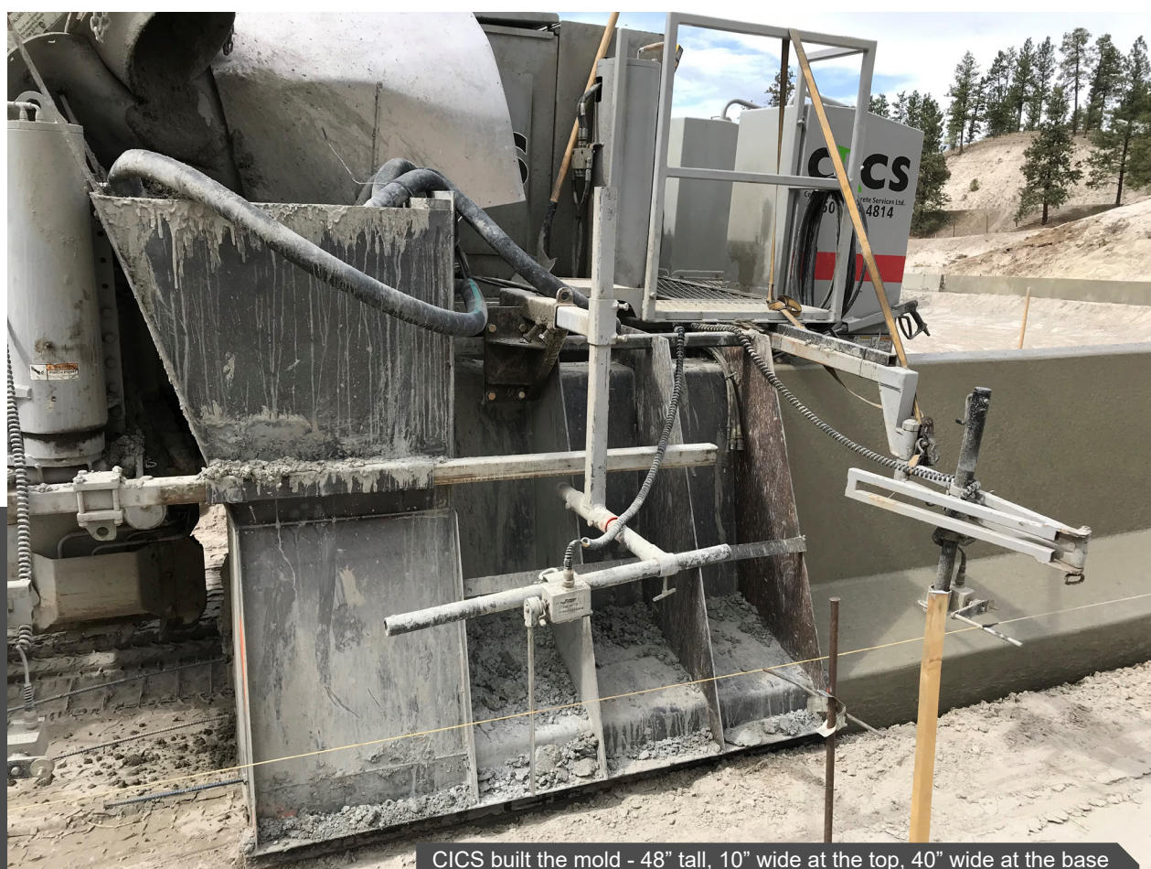
CICS built the mold - 48" tall, 10" wide at the top, 40" wide at the base
